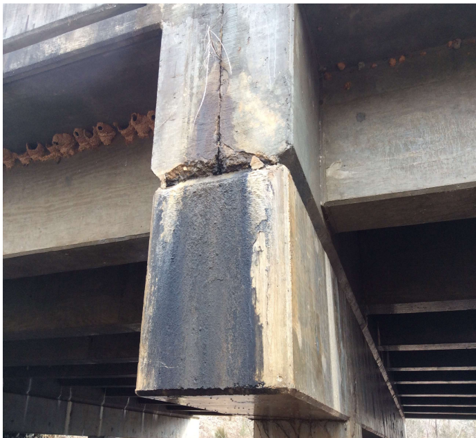
PHOTO 1 Description Spall to Left outside edge of deck at Bent 1.
