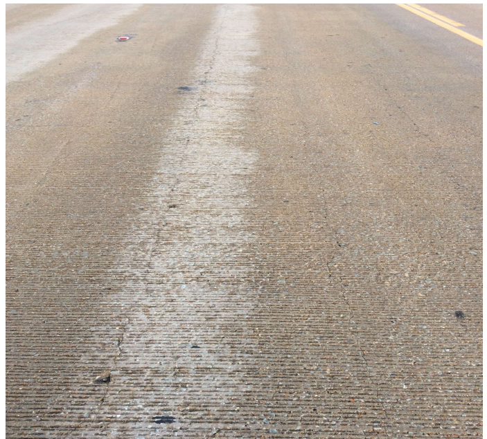
PHOTO 2 Description Typical unsealed cracks to deck at all spans.
